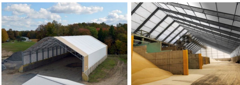
Figure 4: On the right is the I-beam Sidewall style, photo courtesy of Norseman Group Ltd. On the left is the Plate Girder style, photo courtesy of Accu-Steel.
