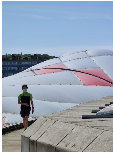
Figure 2. Picture of the Mediacité shopping center roof canopy consisting of ETFE cushions. This structure has been designed by Ron Arad Architects in cooperation with Vector Foiltec GmbH. From the perspective of the room enclosed by the cushions, there is only open air behind the cushions. All the sound energy that passes through the membranes will not be reflected back inside.
