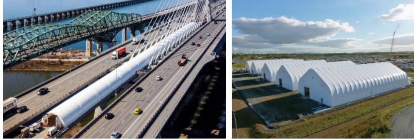
Figure 2: On the left an example of a single cover steel framed building, photo courtesy of Les Industries Harnois. On the right an example of Keder style membrane buildings, photo courtesy of Norseman Group Ltd.
