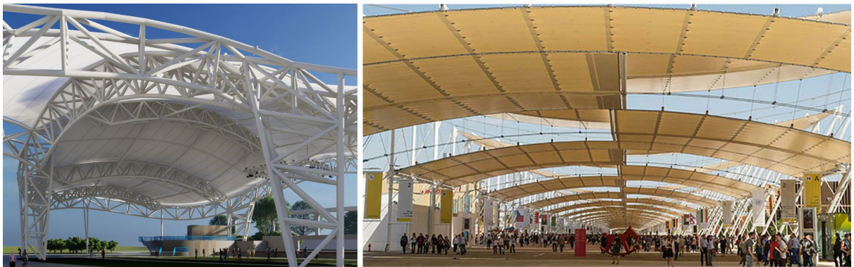
Figure 10: Imagine Clearwater Amphitheater, 2022: the membrane rests on the steel structure. Figure 11: Cardo e Decumano streets, Expo Milano 2015. The membrane hangs from cables. The primary structure is reduced to the lateral masts. Bending is avoided.
