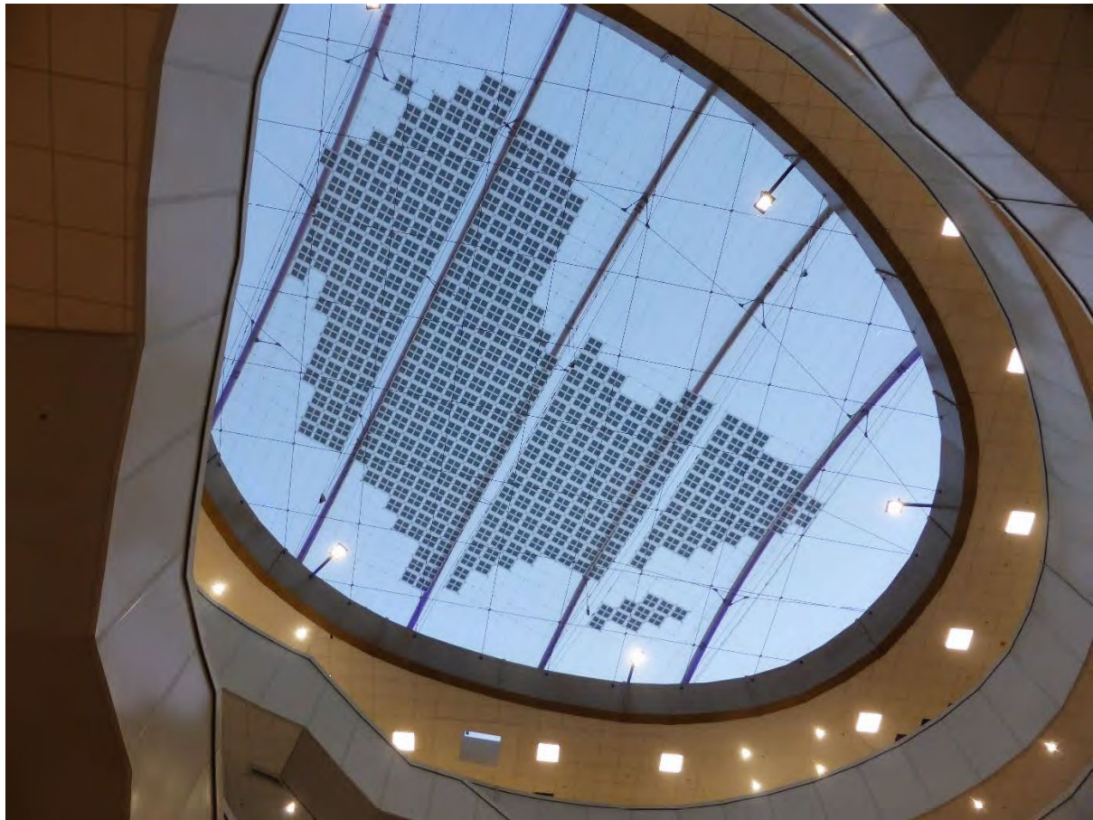
Figure 10: ETFE cushion atrium roof including photovoltaic modules
