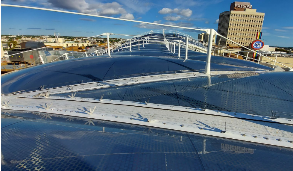
Figure 11: The bluish appearance of the IR-CUT treatment when viewed from the outside, together with the variable surface density screen-printed dots.
