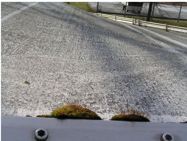
Figure 2a: PTFE/Glass fabric after 11 years
