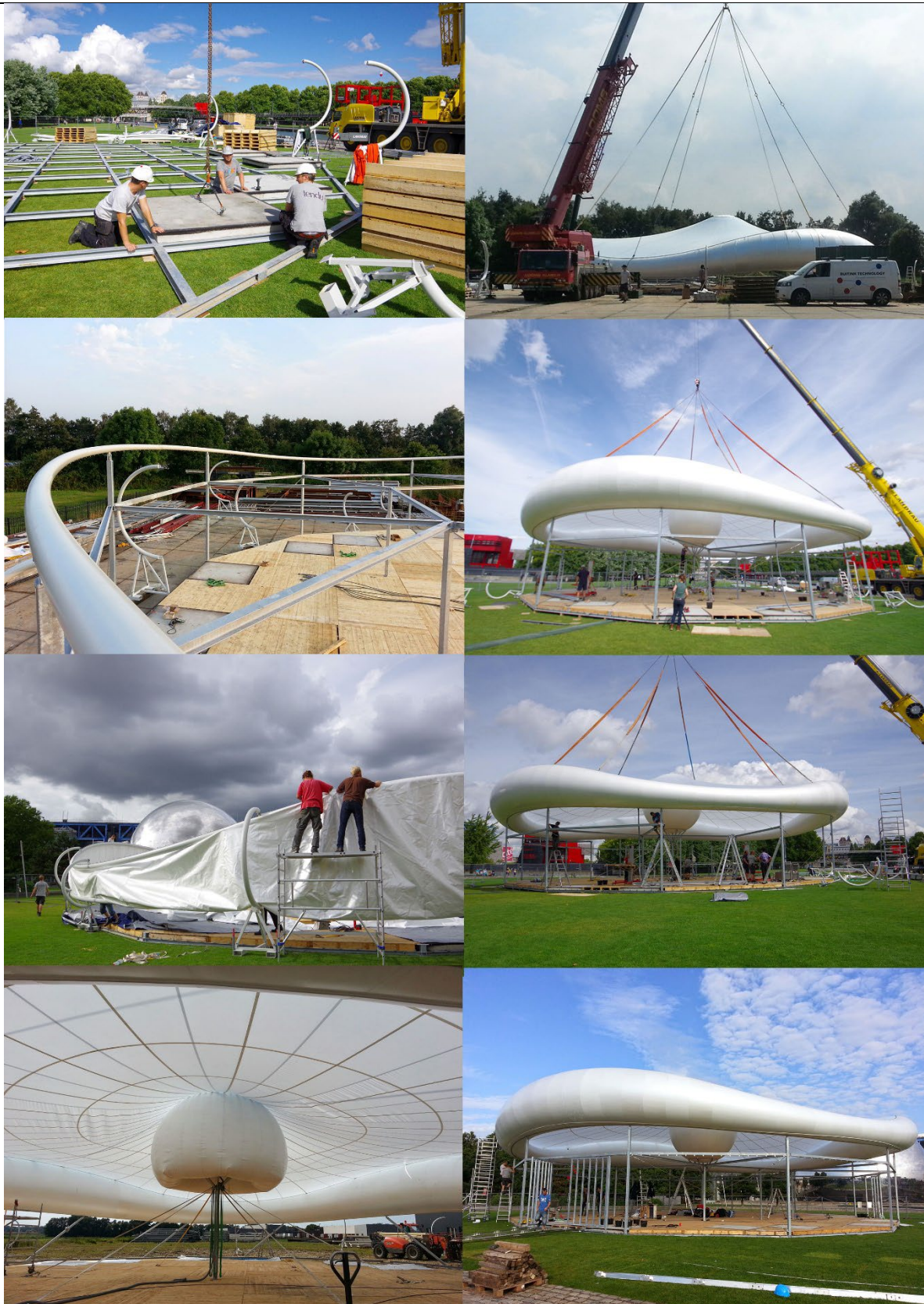
Figure 8: installation of Wave Pavilion structural floor & roof lifted by a crane for supporting structure installation
