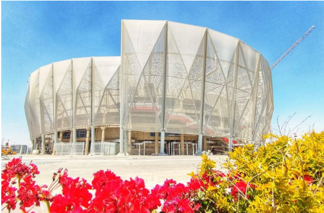
Figure 14: The final look of the facade with the perforated fabric and the visible structure behind
