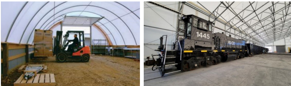
Figure 3: On the left an example of Single Truss building style, photo courtesy of Norseman Group Ltd. On the right an example of Double Truss building style, photo courtesy of GNB Global.
