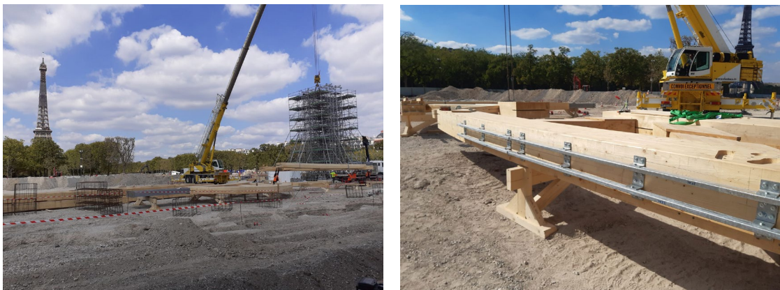
Figure 2: Start on site
