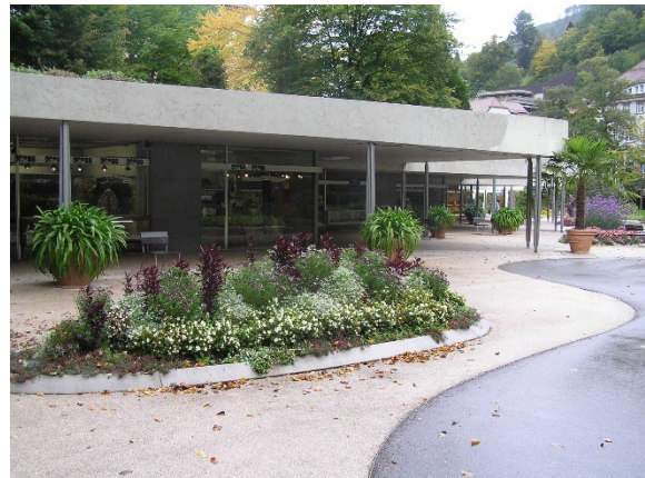
Figure 4b: situation today, removed structure
