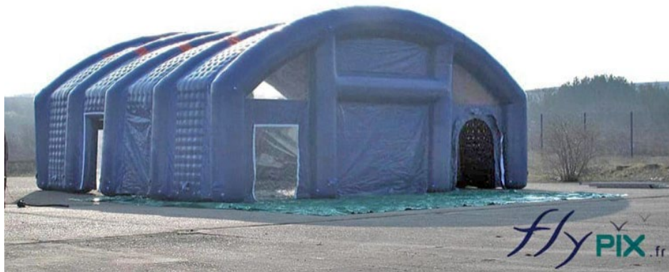
Figure 2: Inflatable structure with tubes, arches and cushion walls with inner threads. (© Vivien Laille, FlyPix.fr)
