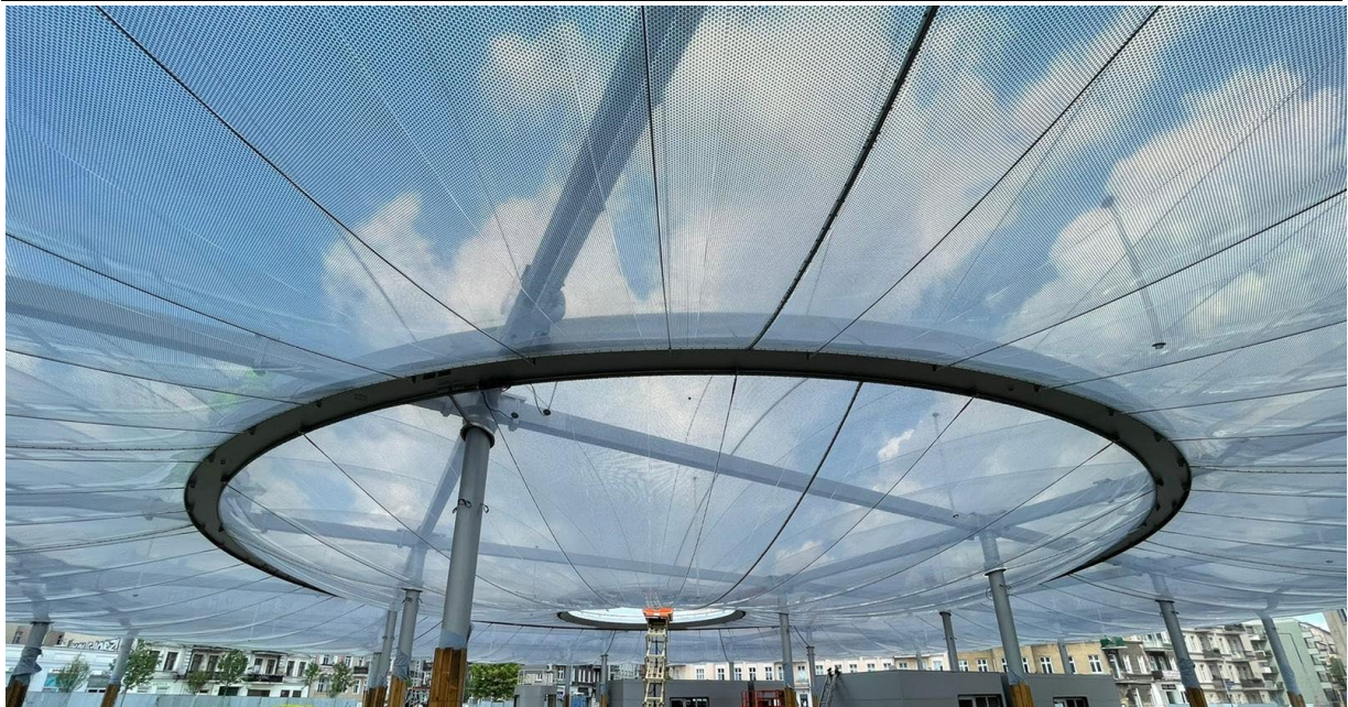
Figure 13: ETFE cushions after installation (source: Temme // Obermeier GmbH)
