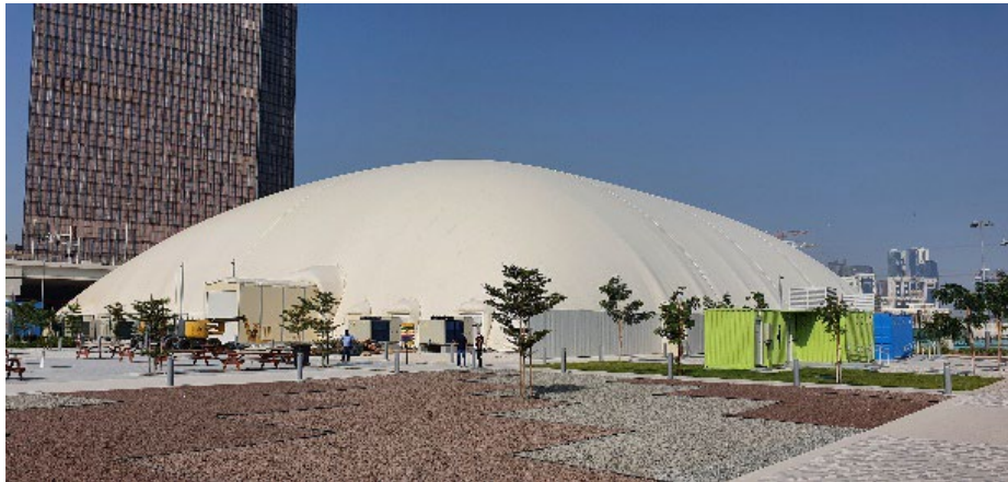
Figure 5: External view of Sports dome Al Maryah
