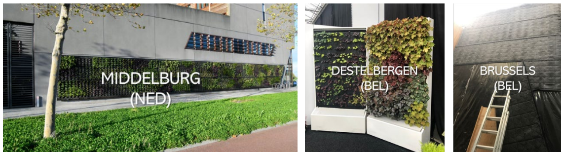
Figure 1: three Greentexx® product and installation types illustrated via three existing projects in Middelburg (with tarpaulin and keder on aluminium profiles), Destelbergen (standard-sized panels with tarpaulin and keder in an aluminium/steel structure), and Brussels (without tarpaulin stapled onto a solid board) (© Sioen Industries)
