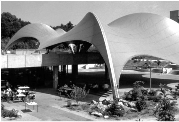
Figure 5a: Textile Cover PH Ludwigsburg, Germany 1980, replacement 2010, (Ref. Institut für Massivbau, University Stuttgart)
